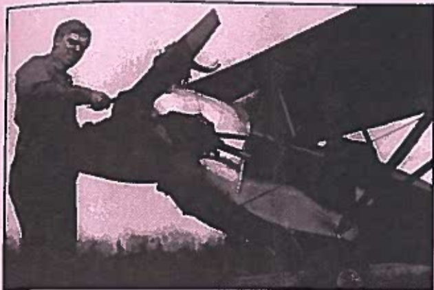
Arthur Shute and Dick Jackson with the Heath Parasol they built in Kennebunkport in 1946. 45 HP 3-cycle Szekeley with 4 inches cut from propeller for ground clearance.
