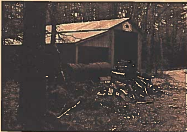
Is this what we're looking for? Hopefully not, for it's a tank boiler from a Lombard steam log hauler.
