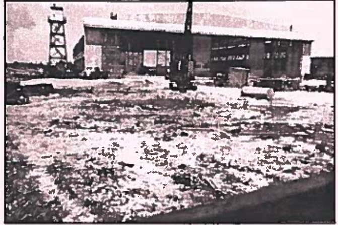
Dow Field, Bangor hangar and tower under construction in 1940. Photo via Al Cormier.
