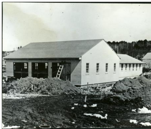
The Bangor Air Base Fire Station Under Construction, Spring 1941
